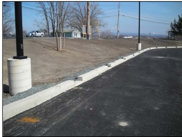
Getting stormwater off of paved surfaces and on to grass/soil areas is an important element of Low Impact Development.
